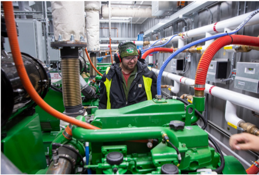
ANTHC engineer Joe Hess examines the power plant (10/24)
